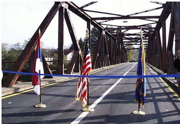
Following the 1992-1995 war in BiH, USAID assistance focused on reconstruction of infrastructure, including major bridges.
